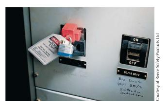
In the case of multiple isolations on a DB, a multilock hasp can be used to prevent access to a main isolator until such time that all persons working on a system have completed their work and removed their padlocks from the hasp.
