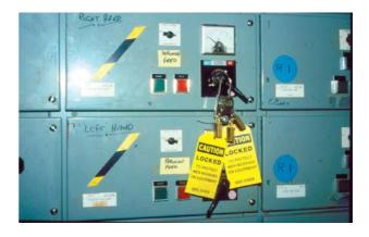
If locking-off facilities are not provided on the relevant switch then a locked DB door or locked switch-room door is acceptable provided the key or combination is unique, and is retained by the person doing the work.
