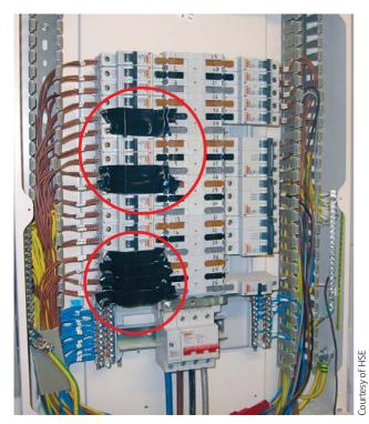
Note: Some DBs are manufactured with 'slider switches' to disconnect the circuit from the live side of the circuit-breaker. These devices should not be used as a means of isolation for circuits, as they do not meet the requirements for isolation and the wrong switch could easily be operated on completion of the work.
