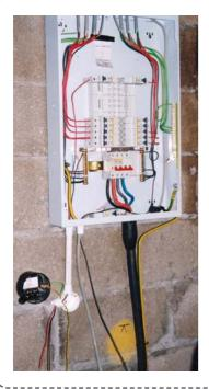
An electrician working on a new-build construction project installed the 3-phase and neutral distribution board shown in the photograph. He energized the supply to the distribution board before the circuits connected to it were complete, to provide a supply to a socket-outlet.
